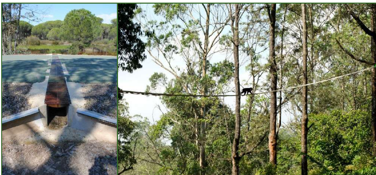
119. Examples of effective habitat linkages across roads. Left: An underpass for reptiles and amphibians in Doñana National Park, Spain [59]. Right: Rope bridges for monkeys and squirrels in India (source: Bridging the Gap by Ganesh Raghunathan)
